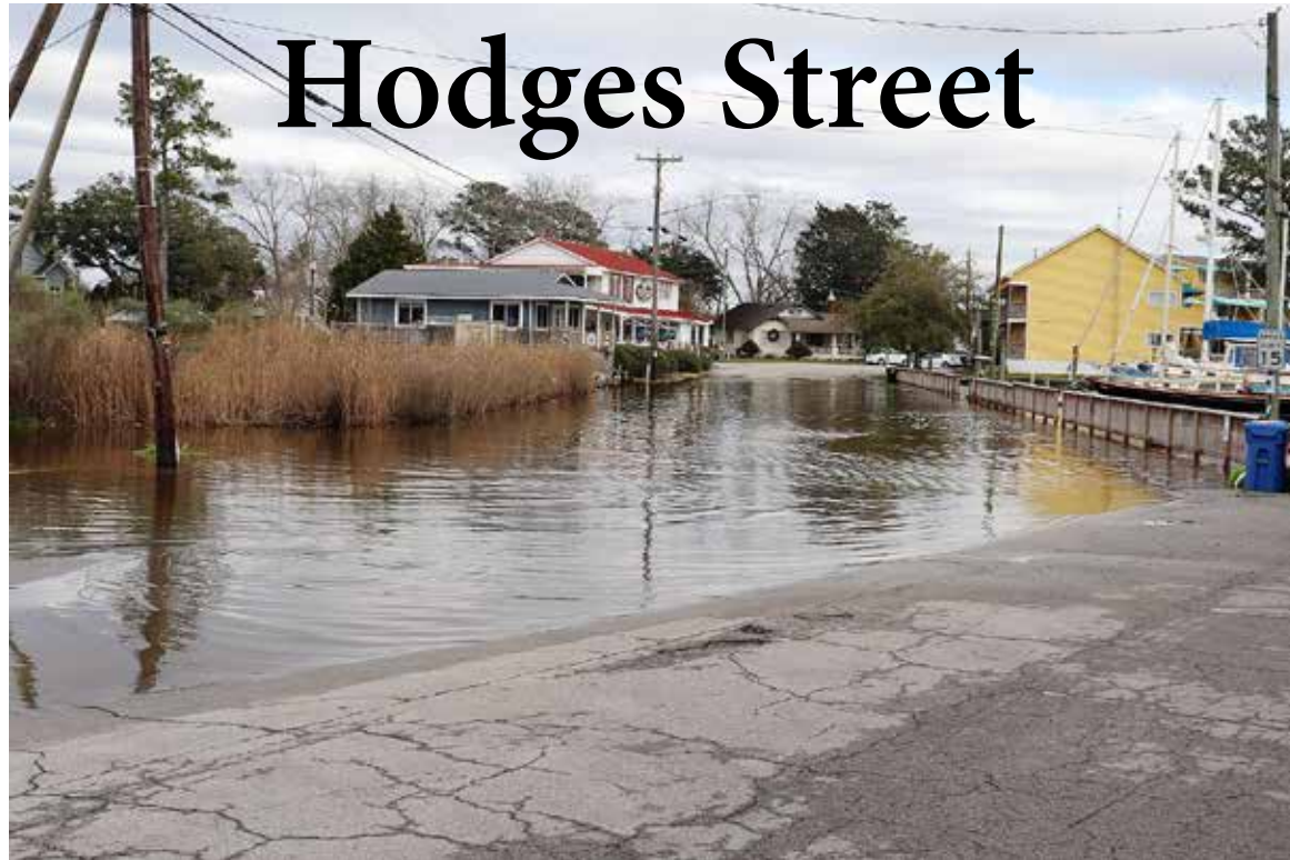
The flood prone area of Hodges Street in Oriental was once again wet Friday as a stiff easterly wind pushed water from the Neuse up into the street.
