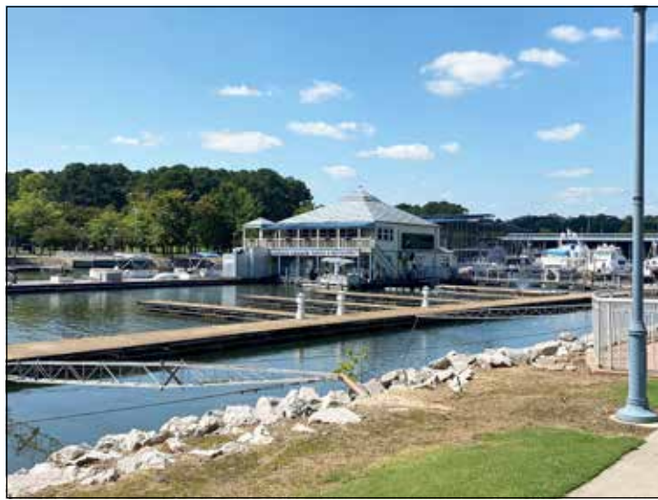
Florence Harbor Marina, Alabama, used BIG funds to renovate an existing 460-foot transient dock by adding new dockside power pedestals, providing water service, and replacing worn decking and flotation. (credit: Alabama Department of Environmental Management)
