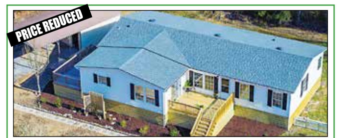
MERRITT – Newly-renovated, 2,100 sf 3BR/2BA , on 1 acre unrestricted lot, no HOA. Home is on an engineered permanent foundation with a HUD Compliant Foundation Engineering Certification letter; qualifies for Conventional, VA, FHA and USDA financing. Roof & HVAC installed 2021. OFFERED AT $305,000
