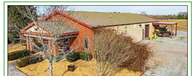
ORIENTAL – 4,000 hsf commercial building on 0.92 acres of unrestricted land, not in flood zone, +/-3 miles north of Town of Oriental. Fully-insulated I-beam construction, 6" concrete floor. Reception area, conference room & 2 offices. Carrier 2.5 ton heat pump for 1,080 hsf office area & two 5.0 ton HVAC systems for 2,920 hsf warehouse. Walk-up attic storage, fenced side yard, 208 3-Phase electrical system with 200 amps service. Ingersoll Rand 200 PSI air compressor system for warehouse with work benches & shelving. Metal fabrication equipment does not convey. OFFERED AT $ 650,000
