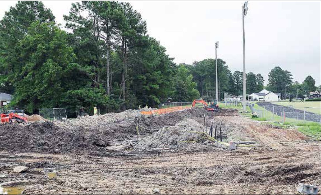
Geothermal well area. After installation, the ground will be leveled, graded, and grassed over and the wells will be invisible above ground.
