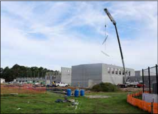
A crane lifts roof beams above what will be the Pamlico Middle School Gymnasium
