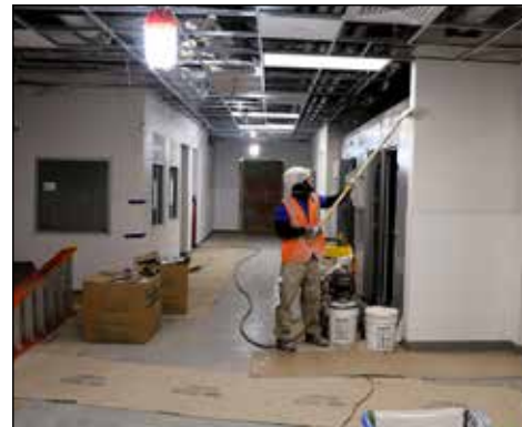
Crewman busy adding paint to walls
