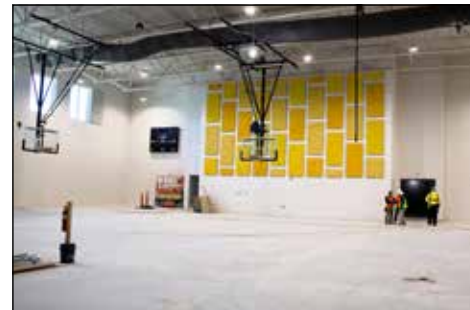
The High School Gym awaiting floor installation
