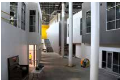
Interior of the new school
