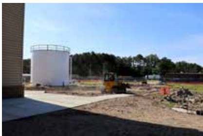
Lot grading behind the new school and the water tank needed for the new school's modern fire suppression system
