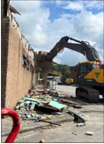
School demolition has started
