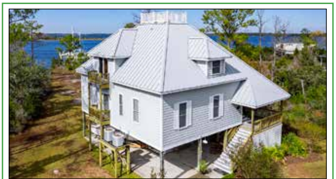
MERRITT – Waterfront 3BR/2BA with deep water deeded boat slip on Ball Creek. Wide water views, 2.27 acres, 1,919 sf, metal roof, zoned HVAC, & LP Smartside exterior for rot-resistant long-life durability. Gas log fireplace in living room, & Widow's Walk with views of the Pamlico Sound, OFFERED AT $ 625,000
