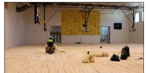
A peek at the new High School Gym. Sanding is being done on the floor before a final top coat and striping are applied and seating is installed.
