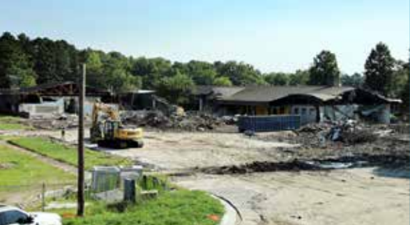
The old school demolition is well over halfway done
