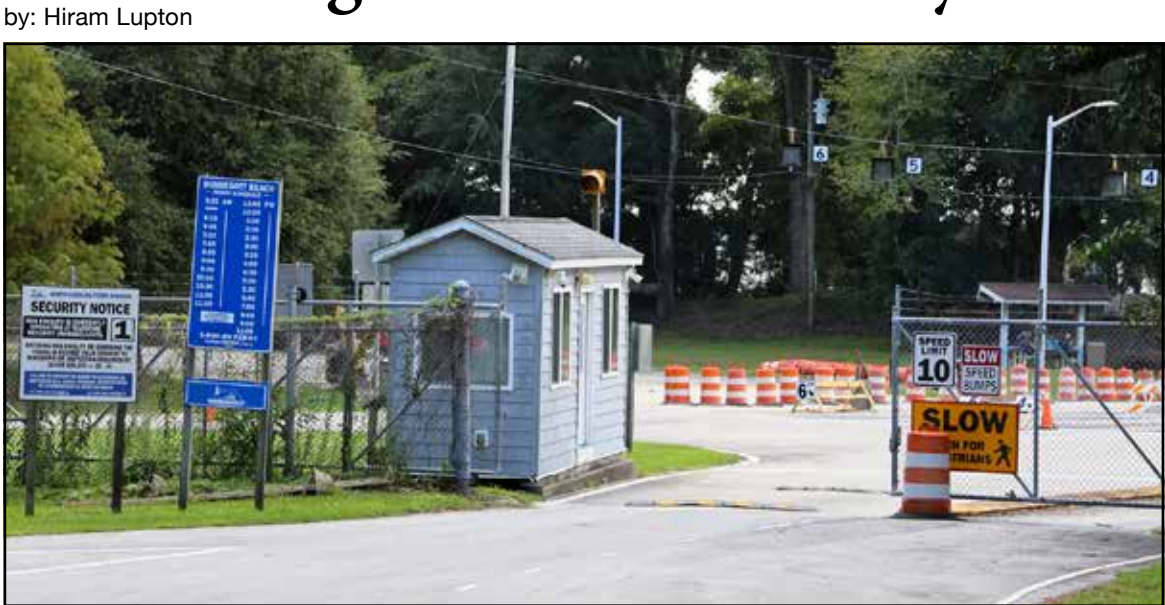
Toll Booths constructed a few years ago when Ferry Tolls were proposed and subsequently defeated may become active on January 1, 2027.
